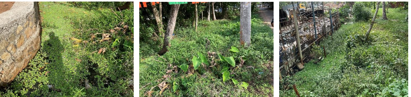
Plate 15: Valiyath Canal (VC-02) located at 0.75 km upstream of the Pallikal River (Lat.: 9° 3'38.09" and Long.: 76°32'23.61")
