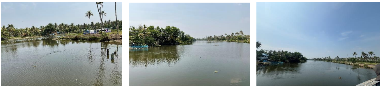
Plate 5: Edappally canal (EC-03) at 7.25km downstream of EC-02 and 0.1km upstream of the Chabakarra canal (Lat.:9°58'51"and Long. 76°20'14")
